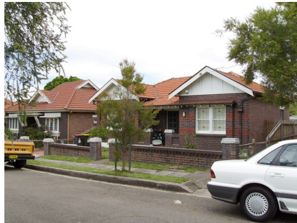
Figure 23.8 All of the houses in the group were constructed of dark red face brick – this house is an unusual example of duo-chrome brickwork used on an Inter-War house, but the patterning is reversed with red banding on dark brick instead of the dark banding on red brick common in the Federation period.
